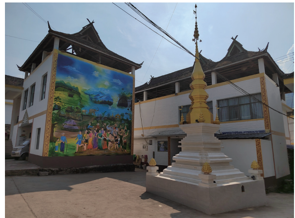
Photo of a rural leisure resort project in Likan, Mengsuo town, Ximeng County
