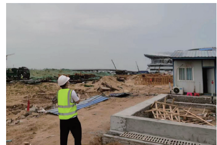
Using drones to inspect the construction site
